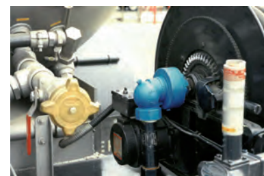
First SMAC hose reel swivel installation
